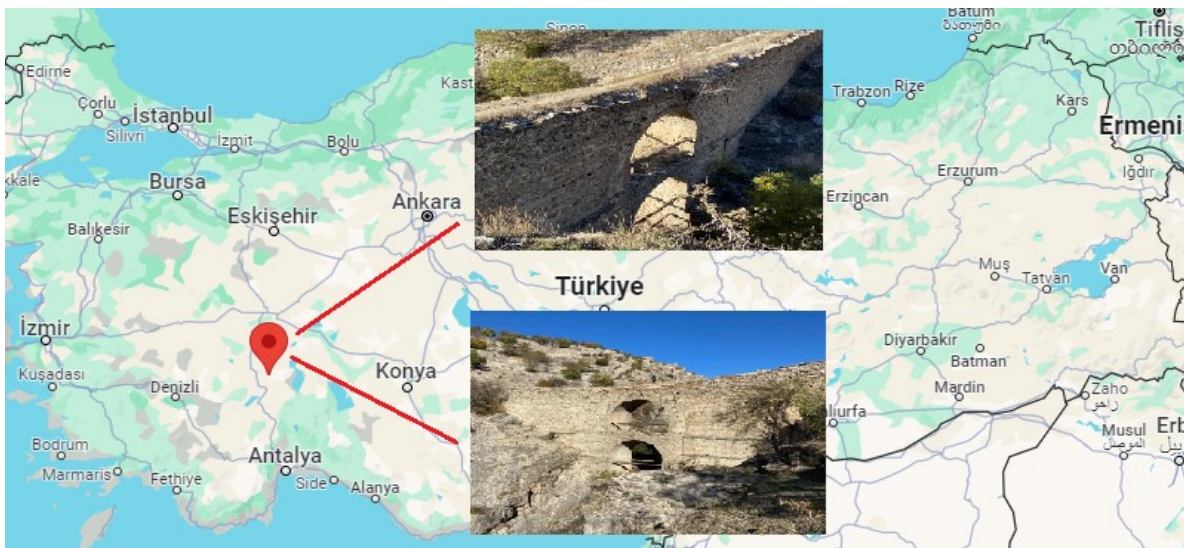
Figure 2: Historical Cirimbolu bridge and its location
