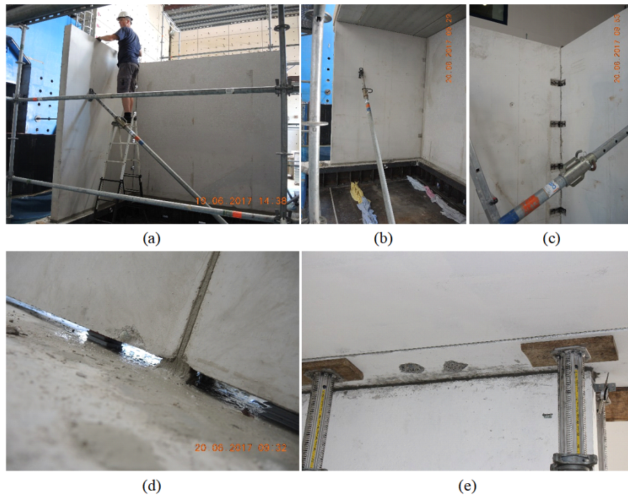
Figure 2: Construction details concerning the installation of precast panels and the execution of mortar joints – adapted from Brunesi et al. [8]
