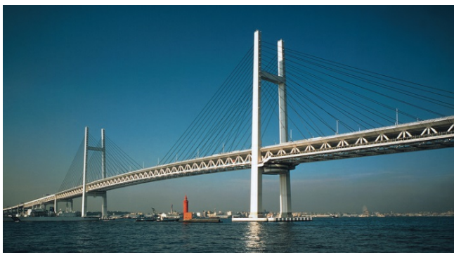
Fig. 6. Yokohama Bay Bridge (source: www.yokogawa-bridge.co.jp/). Ponte Yokohama Bay (www.yokogawa-bridge.co.jp/).
