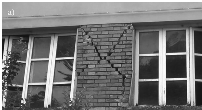
Fig. 13. Column damages. Danni a colonne.
