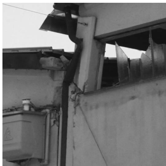
Fig. 13. Column damages. Danni a colonne.
