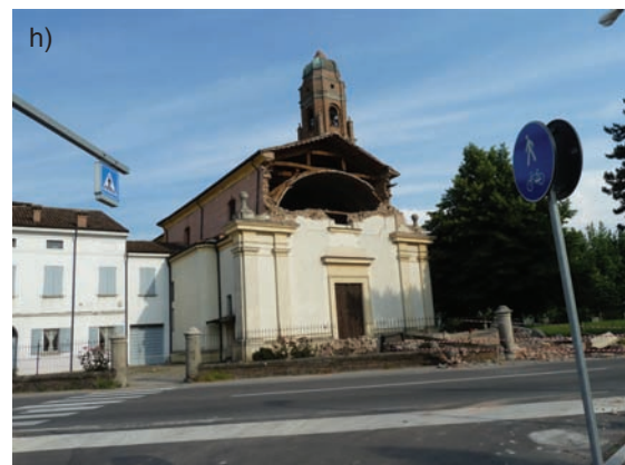
Fig. 33. The incurred damage of churches follows almost an identical pattern. The bell towers survived with only minor damage along the height. In most cases the top of the spire was damaged; a), b) church of San Marino at Buonacompra; c), d) church of San Francesco at Mirandola, very heavy damage. The bell tower collapsed after the second event; e) Santa Maria Maggiore, Cathedral of Mirandola; f) a view from the north towards S-E; g), h), two damaged churches in Mirandola.
