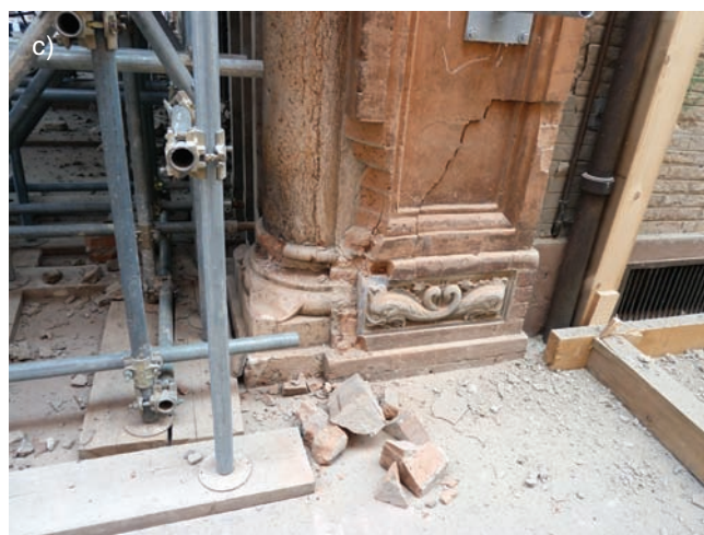
Fig. 26. The Mirandola Town hall; a) no major damage is noted by a rapid optical survey from the exterior, except the damage shown in b) and c) at the bottom of the masonry columns due to impact.
