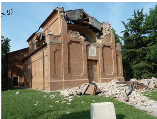
Fig. 33. The incurred damage of churches follows almost an identical pattern. The bell towers survived with only minor damage along the height. In most cases the top of the spire was damaged; a), b) church of San Marino at Buonacompra; c), d) church of San Francesco at Mirandola, very heavy damage. The bell tower collapsed after the second event; e) Santa Maria Maggiore, Cathedral of Mirandola; f) a view from the north towards S-E; g), h), two damaged churches in Mirandola.
