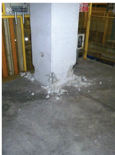
Fig. 25. a) A reinforced concrete structure, in Sant' Agostino ceramic factory, the only recorded damage was around the base of almost all its internal columns; b) There is no shortening of the column at the point of impact. Apparently the damage was caused by tension. Due to this tension the intensity of the impact is augmented, because of the stored energy in the reinforcement.
