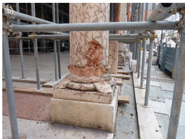
Fig. 26. The Mirandola Town hall; a) no major damage is noted by a rapid optical survey from the exterior, except the damage shown in b) and c) at the bottom of the masonry columns due to impact.
