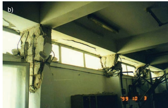
Fig. 28. A part of a wall with a "short column". The pressure p (kPa) due to vertically propagated body waves, integrated along the length ( l ) produces a force F of an impact character. The residual shortening of height ( h ) is relatively extremely small.
