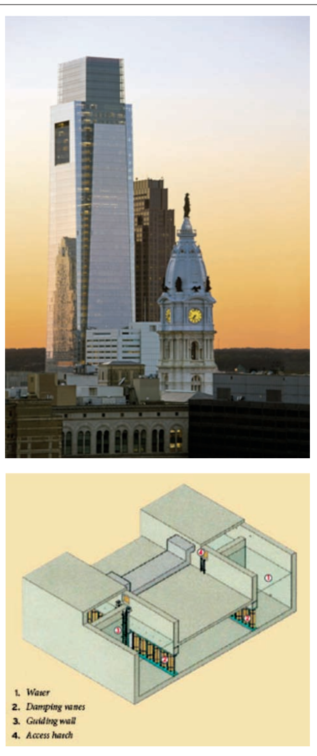
Fig. 12. Comcast Centre view and a 3-D rendering of the TLCD designed and implemented.
