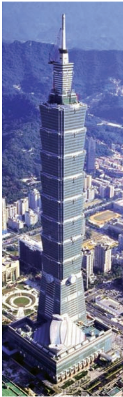
Aerial view of the building
