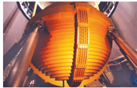
TMD after completion
