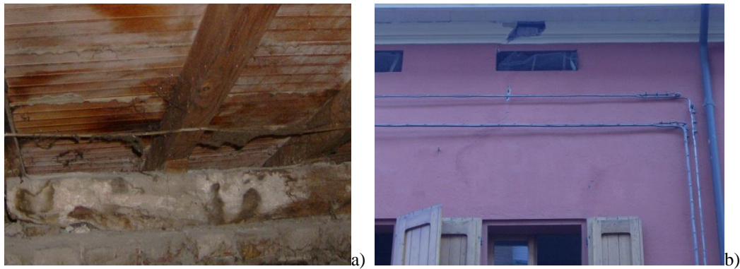
Figure 18: a) Typical timber plate found at roof level in the historic center of Cento and b) out of plane of the related façade due to the discontinuity of the timber plate.
