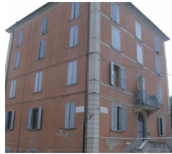
Figure 19: Typical quoins on both edges of the façades. The building on the corner between Guglielmo Marconi street and Costa street in Crevalcore suffers of shears on the spandrels.
