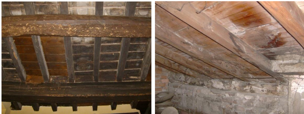
Figure 10: Timber floor and timber roofs inspected in a typical buildings in Emilia Romagna region.
