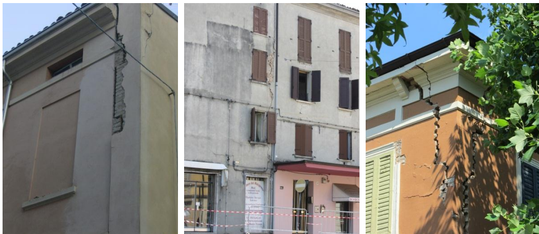
Figure 15: Examples of out of plane in the historic center of Mirandola.
