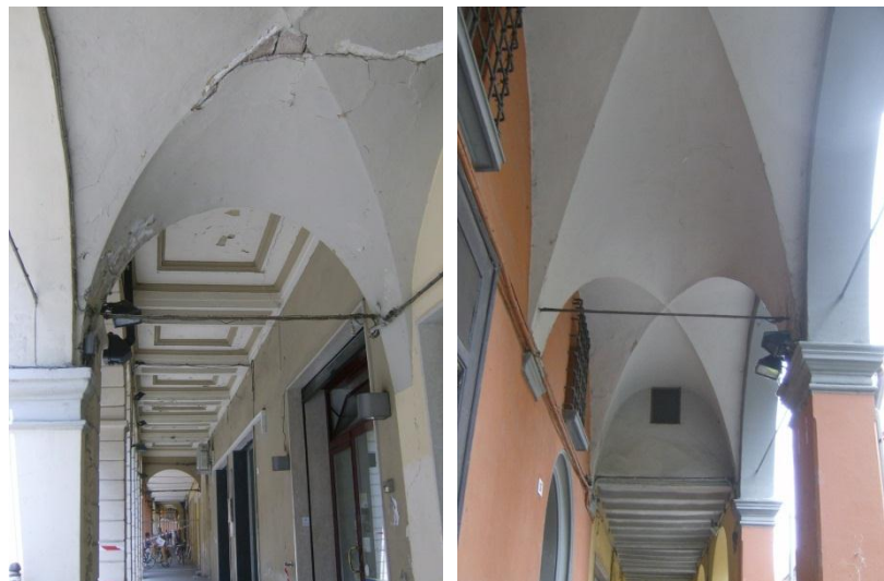
Figure 11: Masonry vaults supported by porticoes observed on the ground floor of the buildings.
