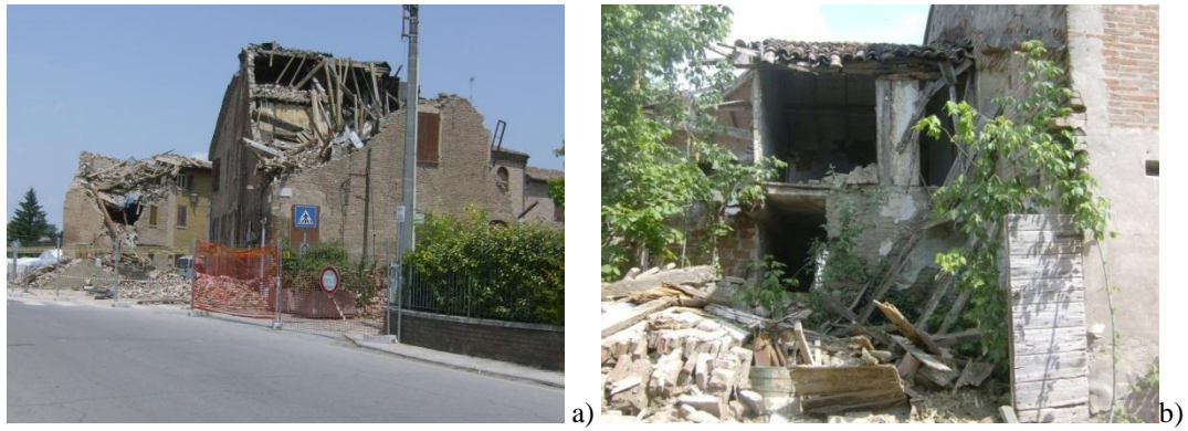
Figure 7: a) Isolated houses between S. Felice sul Panaro and Rivara and b) Isolated house in the neighbourhood of Casumaro characterised by low quality of materials and mortar.
