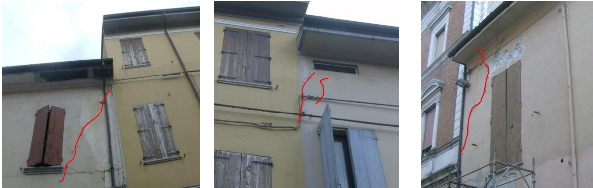
Figure 5: Pounding effect due to different heights of buildings in the historic center of Cento.
